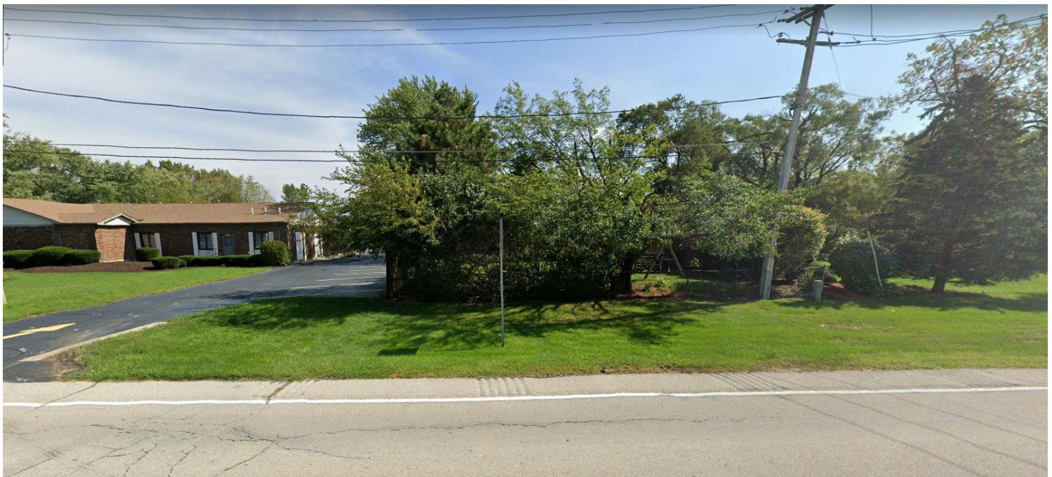
Above: Looking east at the subject property and Kingdom Hall of the Jehovah's Witnesses from Ridgeland Avenue.
